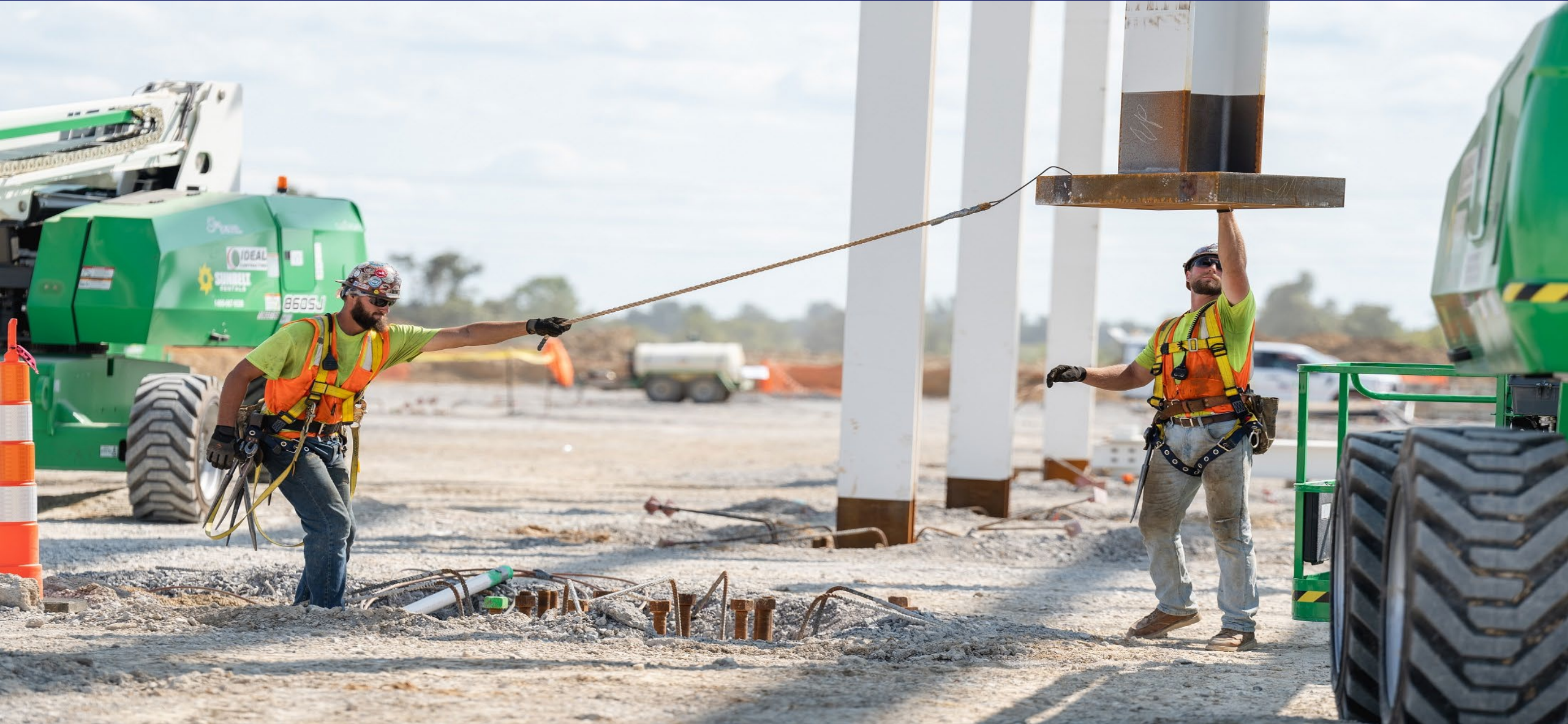
Structural Steel Is Erected At BlueOval City In Tennessee
